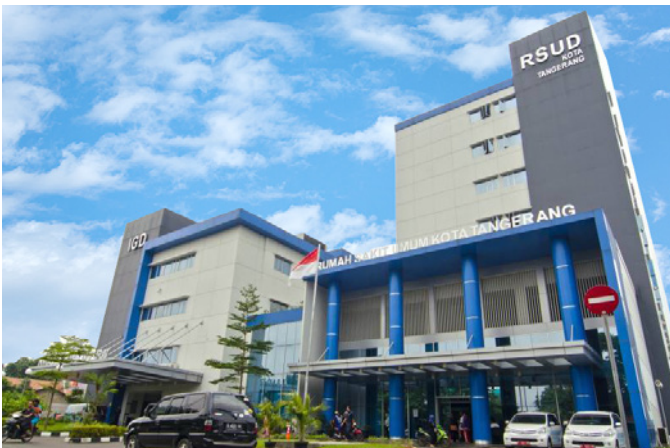
RSUD Kota Tangerang Isolation Transformer
