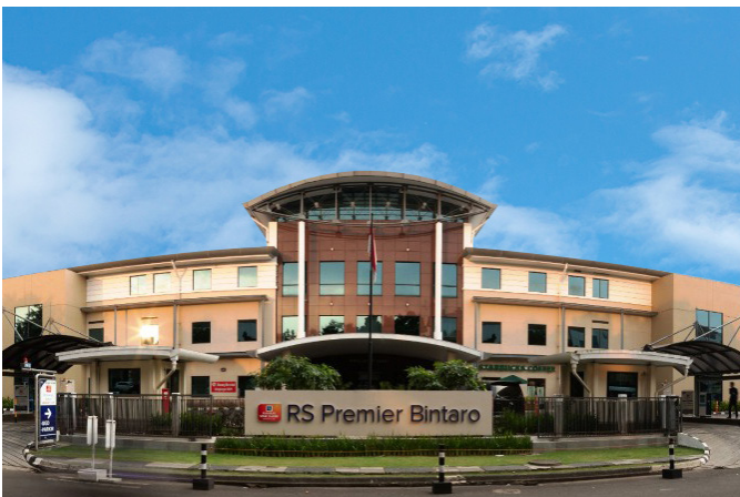
RS Premier Bintaro Isolation Transformer
