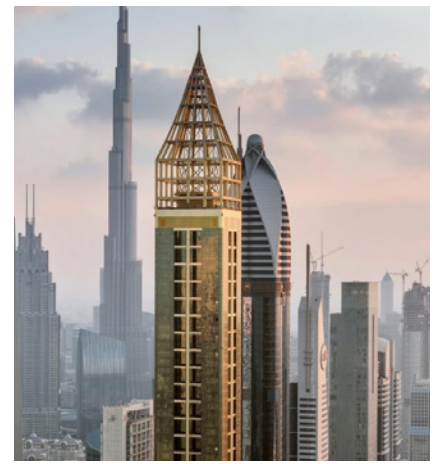
Gevora Hotel, Dubai Guest rooms. Lighting, AC, Shading
