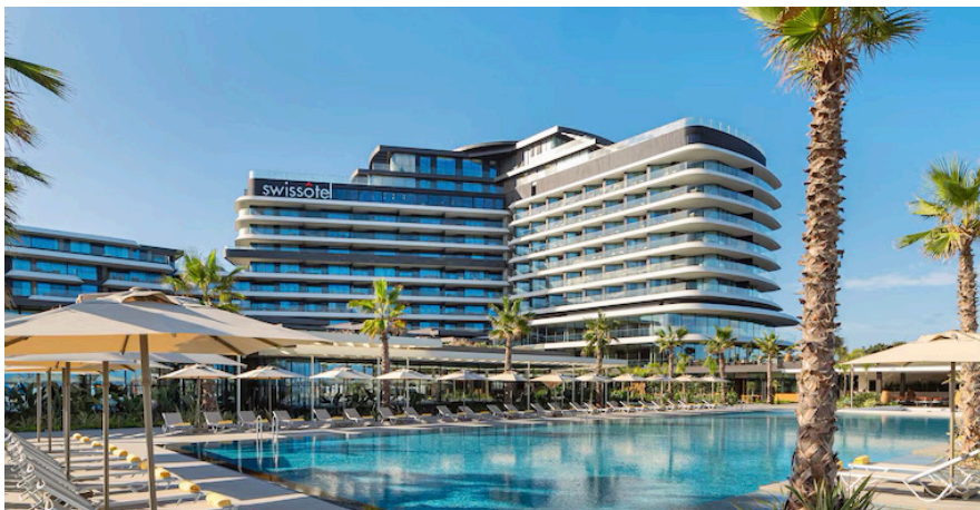
Swissôtel Resort & Spa, Turki Lighting & dimming control, thermostat and sensors
