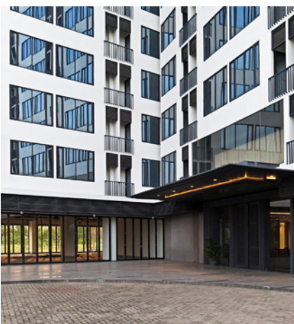
One Narita Residence, Tangerang Lighting control at lobby
