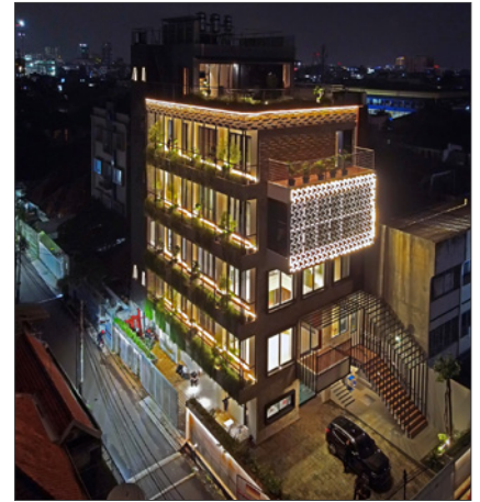
Infotech Office Building Lighting, AC, Blind, Sensor, App
