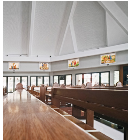
St. Monica Church BSD, Serpong DALI lighting control
