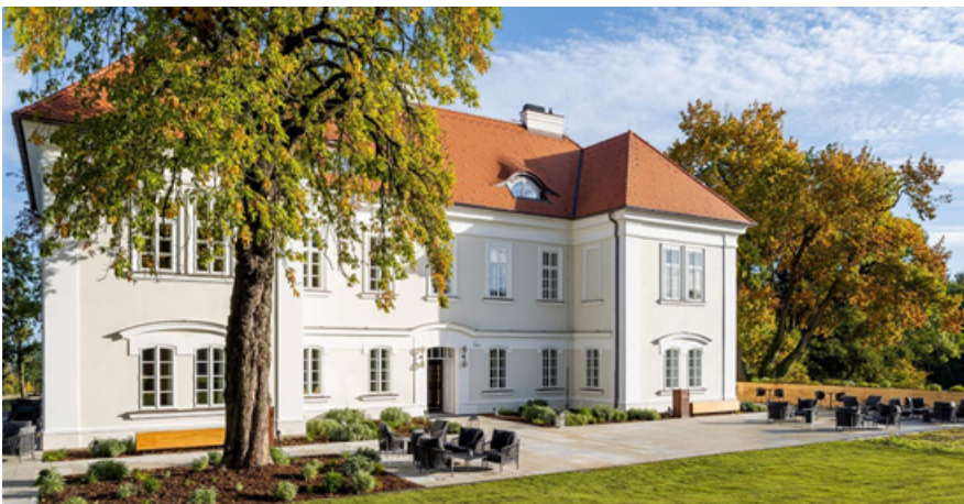
Nebřenice Castle, Czech Lighting and Dimming control, Scenes, Sensors and HVAC control
