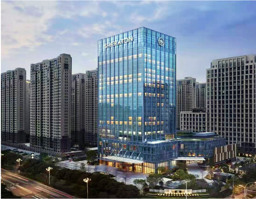
Sheraton Fuqing Hotel, China 348 guest rooms. Lighting, AC, Curtain and Scenes control
